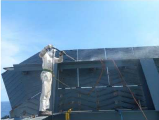
Surface preparation - high pressure water
