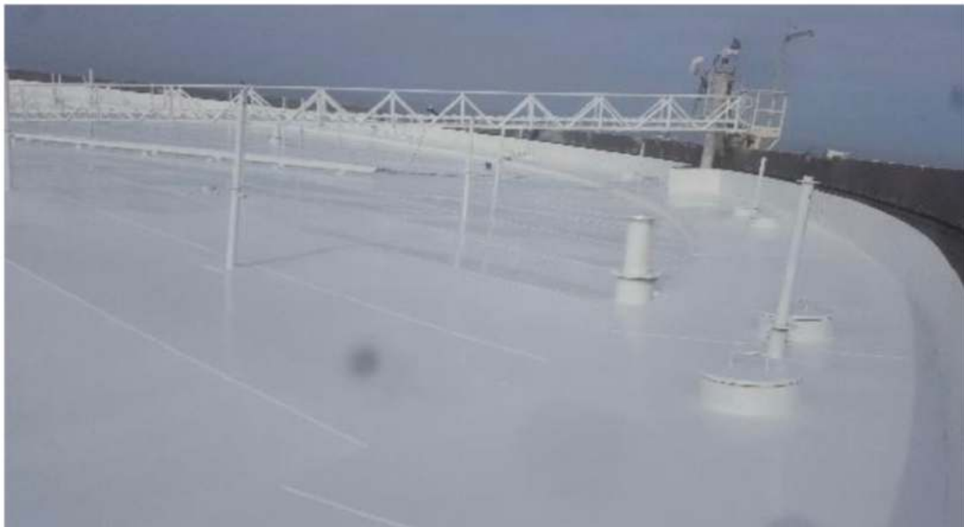
Floated roof appearance after polyurethane top paint
