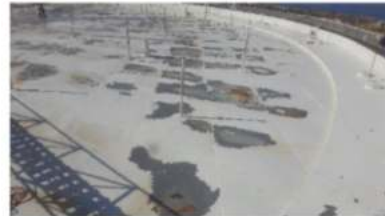
Floated roof initial condition
