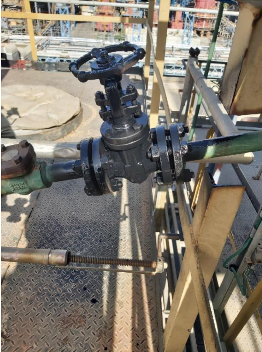
4. Faucet on facility 136
