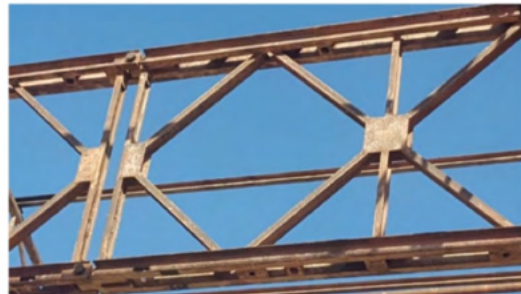
Warehouse's complexity element
