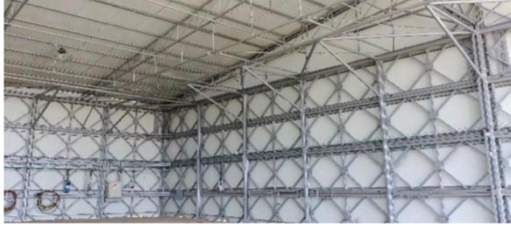
shed condition after treatment
