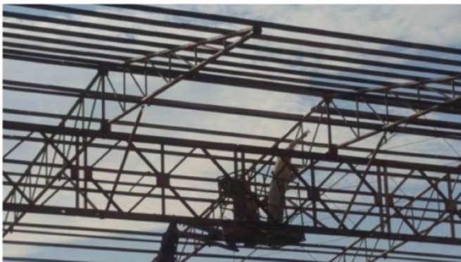
Single layer application with Airless
