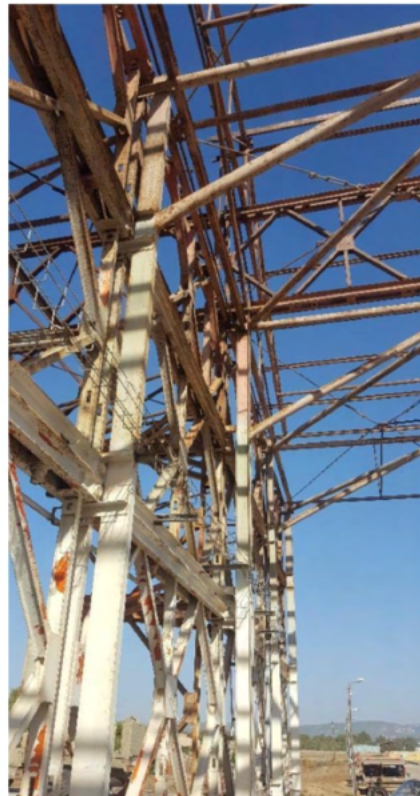
shed condition before treatment
