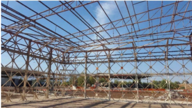
shed condition before treatment
